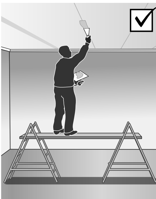
Figure 26 (b) A safer alternative: plasterers' trestles
