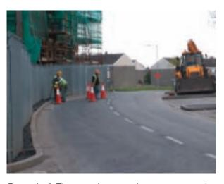
**Example 2** Three workers carrying out construction work at busy bend on roadway. Insufficient and inadequate signing, lighting and guarding measures in place to protect the work crew and other road users.
