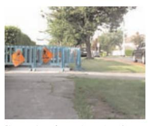
**Photograph 12** Construction work on footway; access around the footway for users is on the grass margin a safe distance from the roadway.
