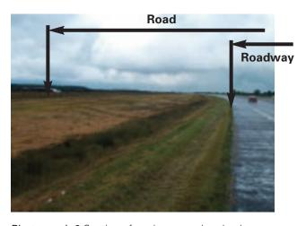
**Photograph 2** Section of carriageway showing how the road can extend way beyond the roadway.
