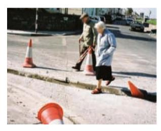
Example 1 Inadequate protection of this construction work on the roadway, resulting in elderly road users having to step over an open trench. Adequate signing, lighting and guarding measures should have been implemented to prevent this situation occurring.
