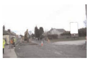
**Photograph 9** Roadway open at busy junction; available width of road reduced; no traffic management plan in place.
